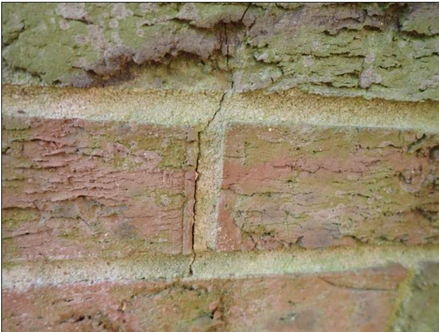
Photo 10 Step crack
