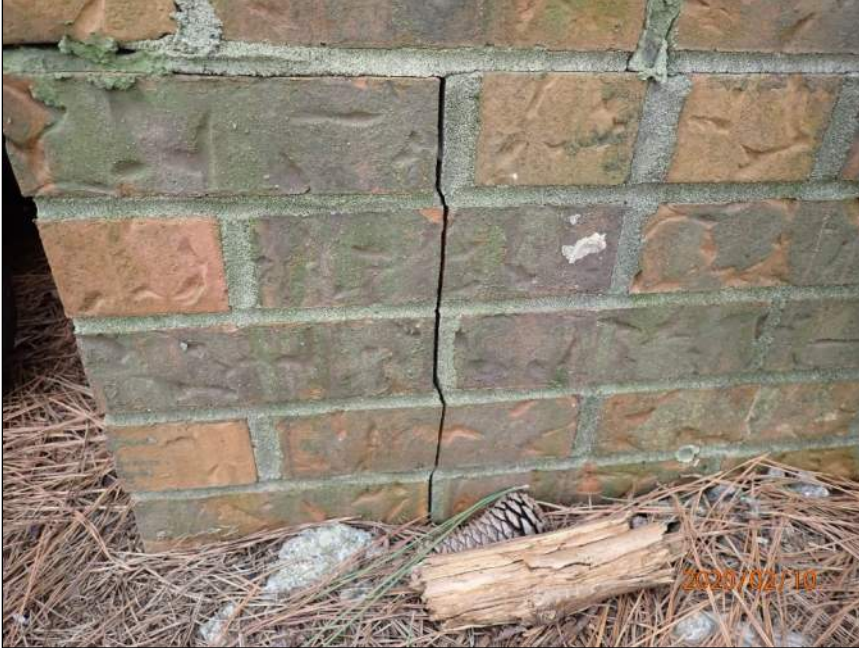
Photo 7 Vertical crack
