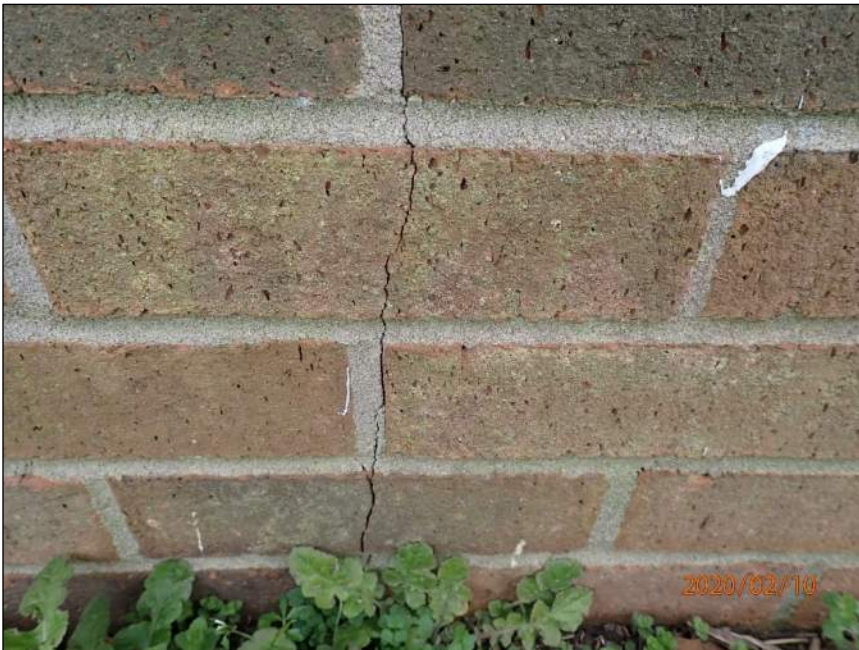
Photo 10 Vertical crack
