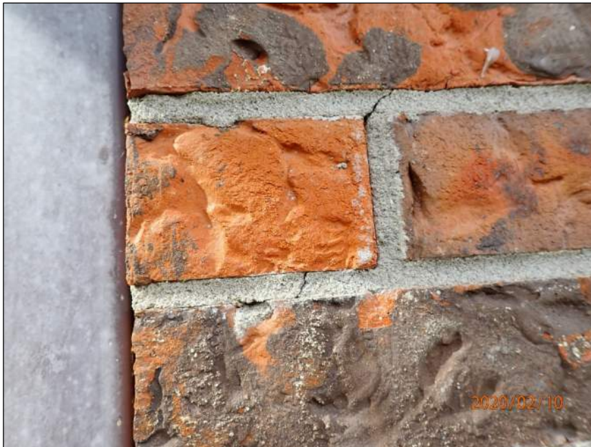
Photo 10 Step crack
