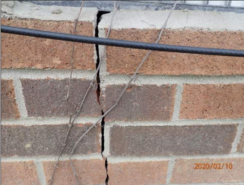
Photo 15 Step crack
