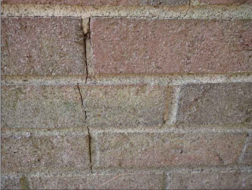
Photo 9 Step crack
