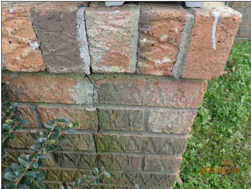
Photo 8 Vertical crack
