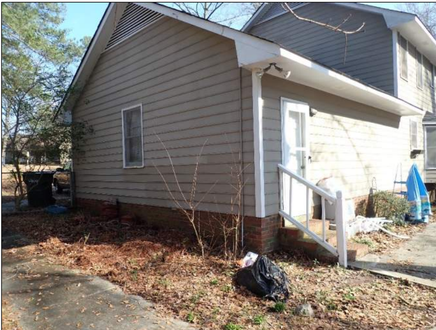
Photo 4 Area of residence observed – side elevation
