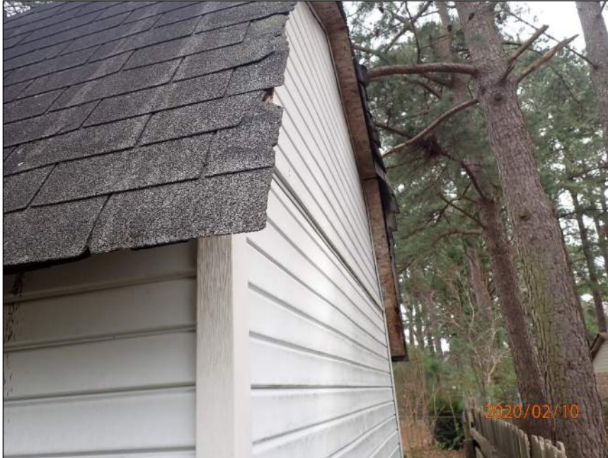
Photo 3 Area of structure observed
