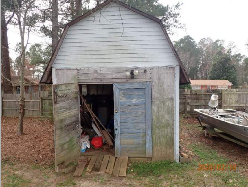
Photo 1 Area of structure observed
