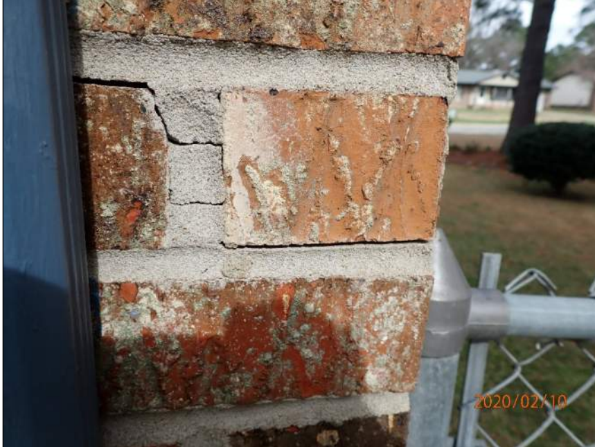
Photo 11 Step crack
