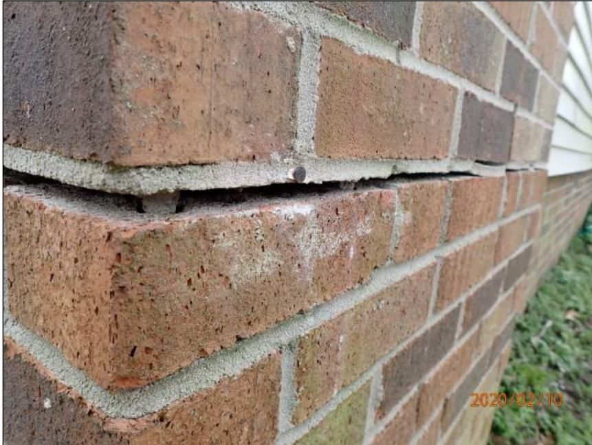
Photo 7 Horizontal crack
