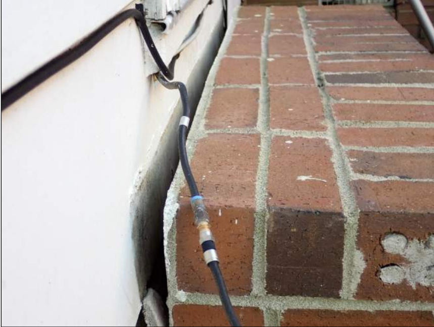
Photo 13 Separation crack
