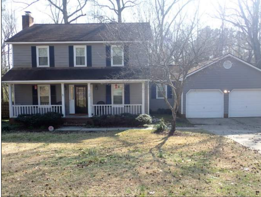
Photo 1 Area of residence observed – front elevation
