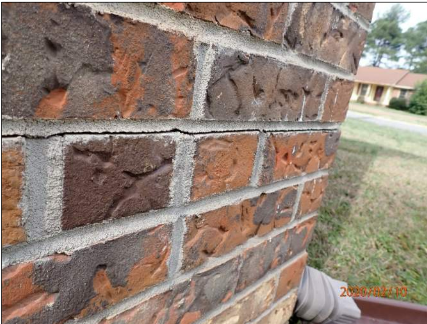
Photo 12 Horizontal crack
