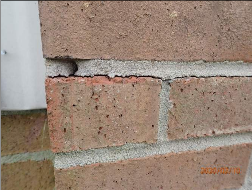
Photo 11 Horizontal crack
