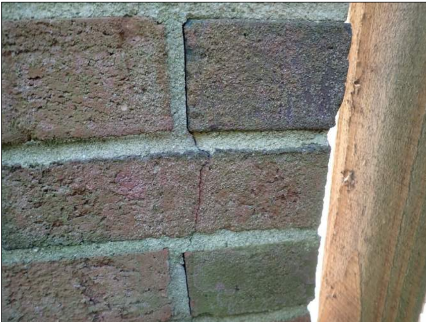
Photo 12 Vertical crack
