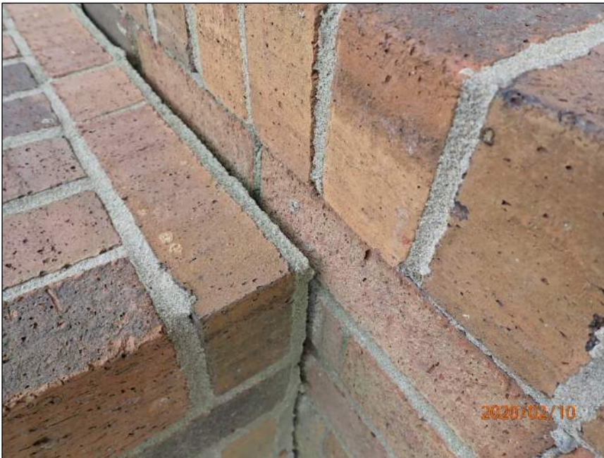
Photo 12 Separation crack
