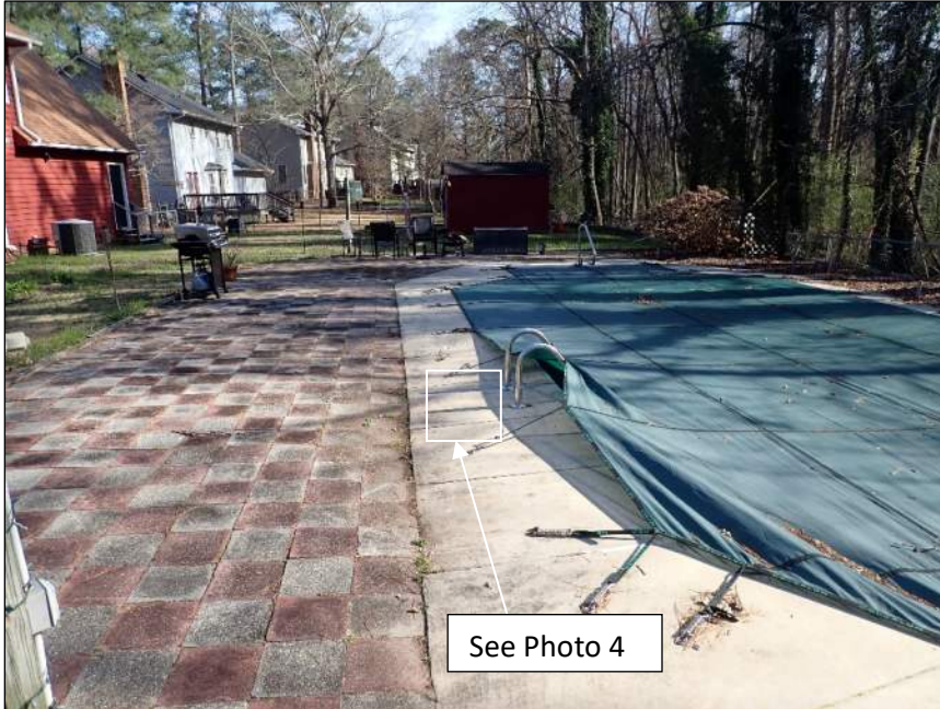
Photo 3 Area of pool observed
