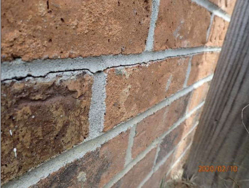
Photo 9 Horizontal crack
