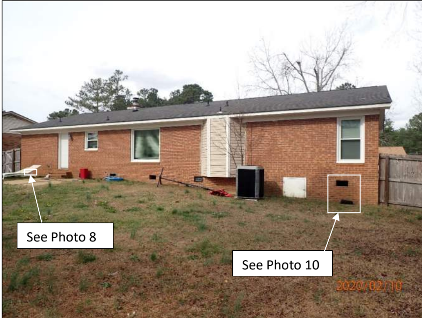
Photo 3 Area of residence observed – rear elevation
