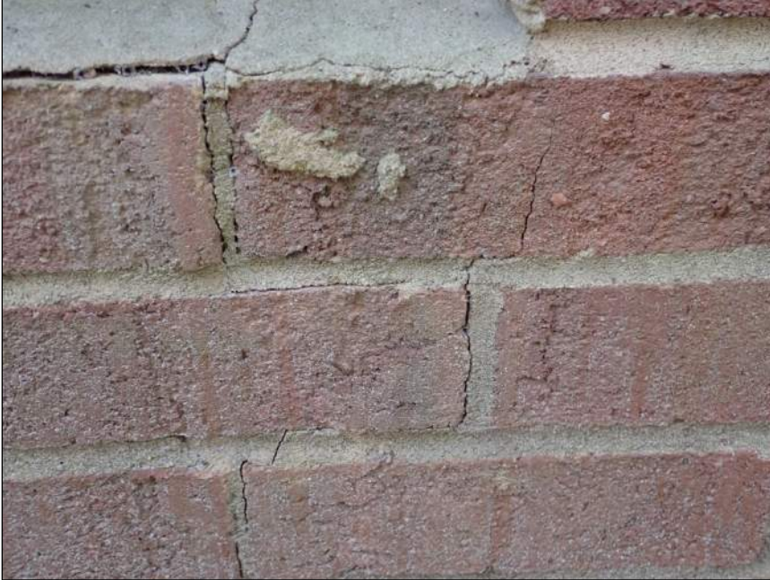
Photo 9 Step crack
