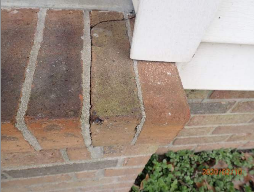
Photo 13 Separation crack
