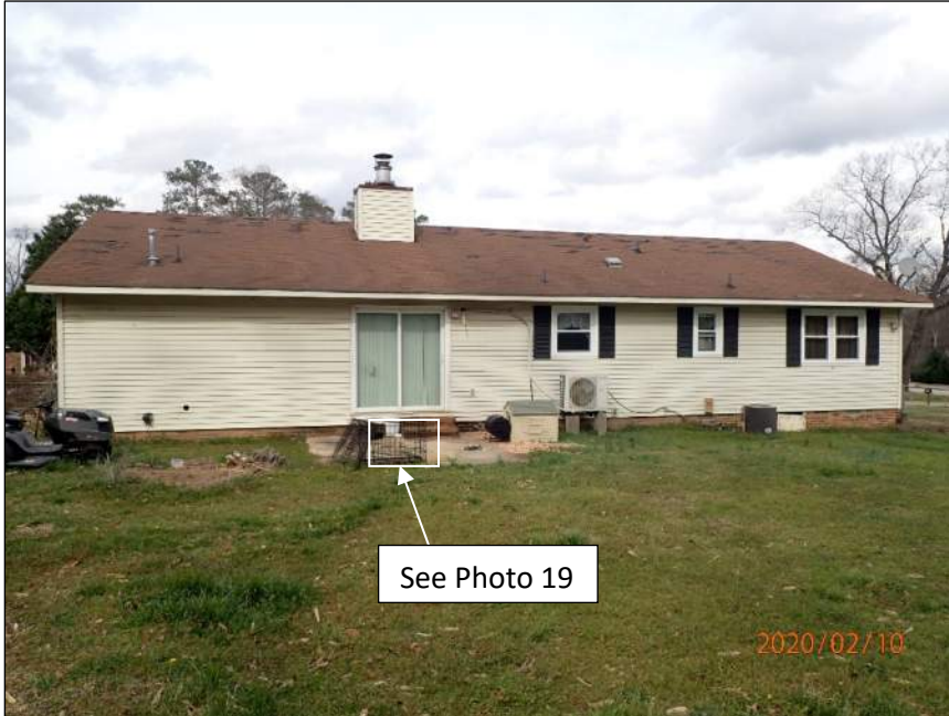
Photo 3 Area of residence observed – rear elevation
