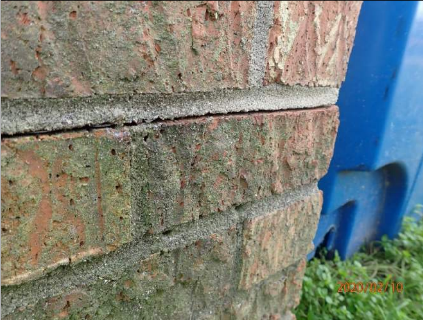
Photo 9 Horizontal crack
