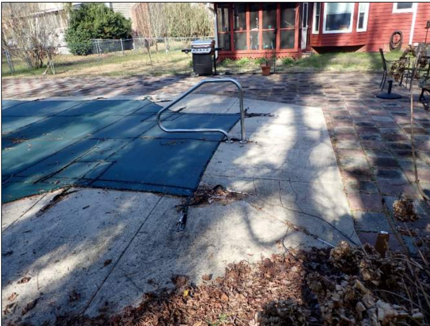
Photo 2 Area of pool observed
