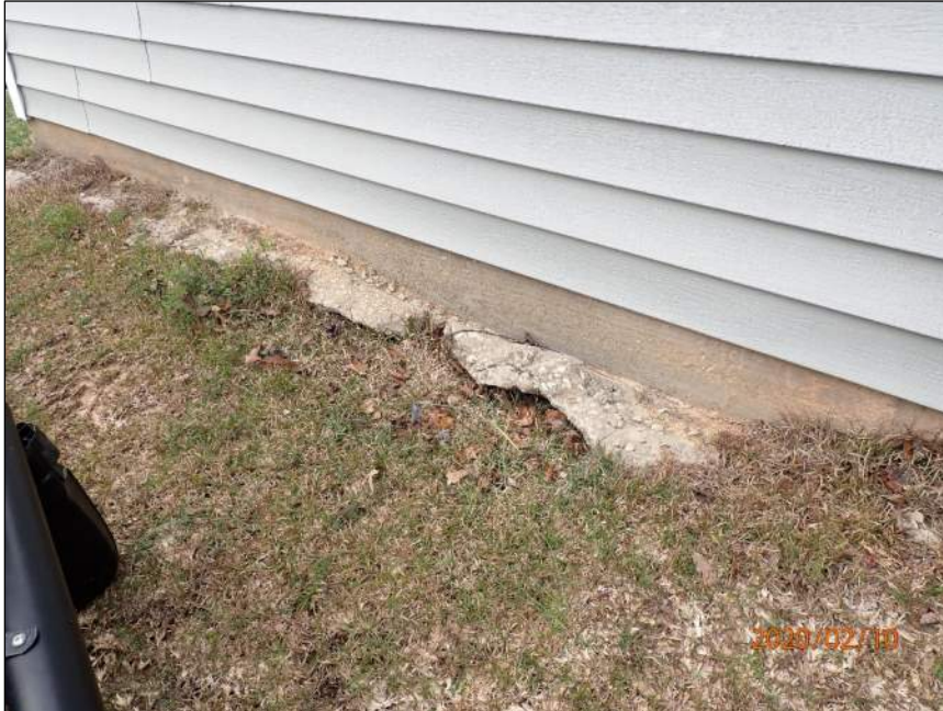
Photo 5 Undermined foundation
