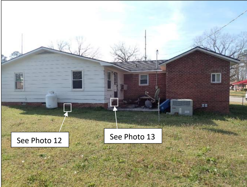
Photo 3 Area of residence observed – rear elevation
