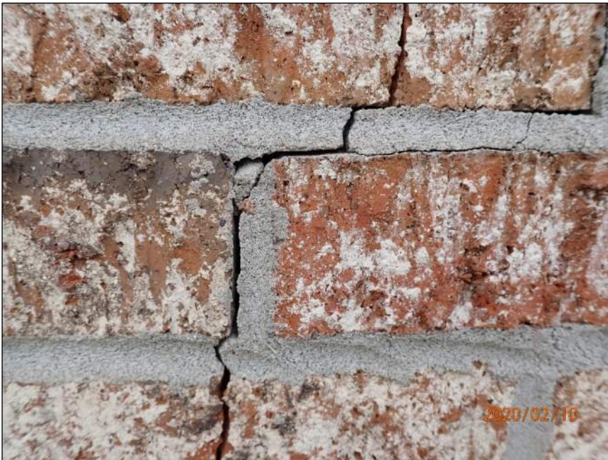
Photo 10 Step crack
