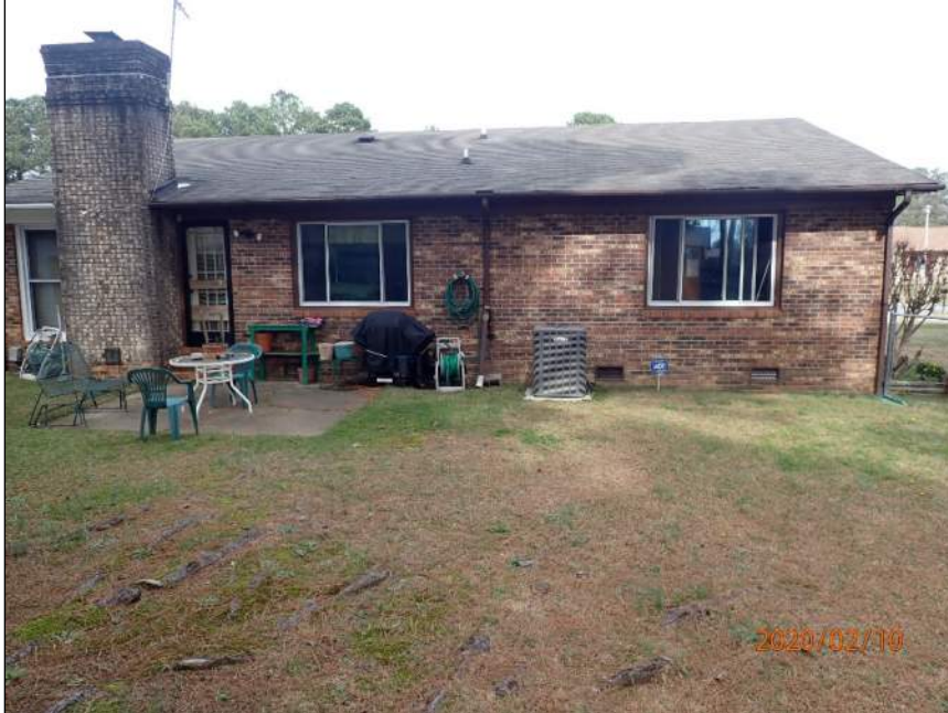
Photo 3 Area of residence observed – rear elevation
