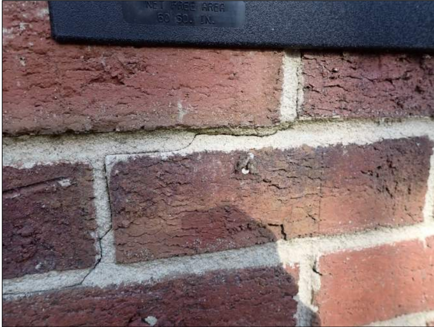
Photo 11 Step crack
