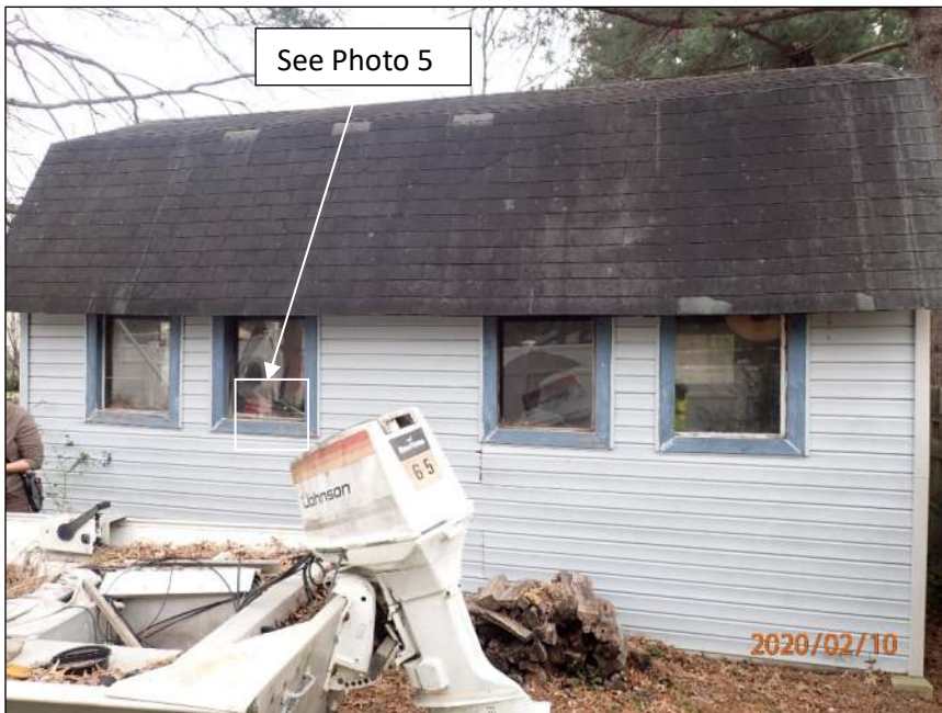
Photo 4 Area of structure observed
