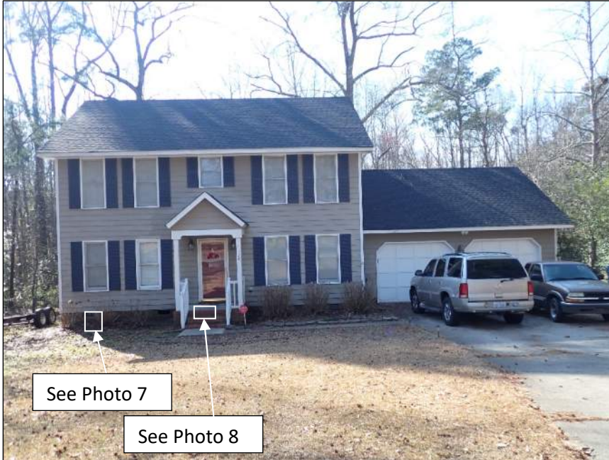
Photo 1 Area of residence observed – front elevation
