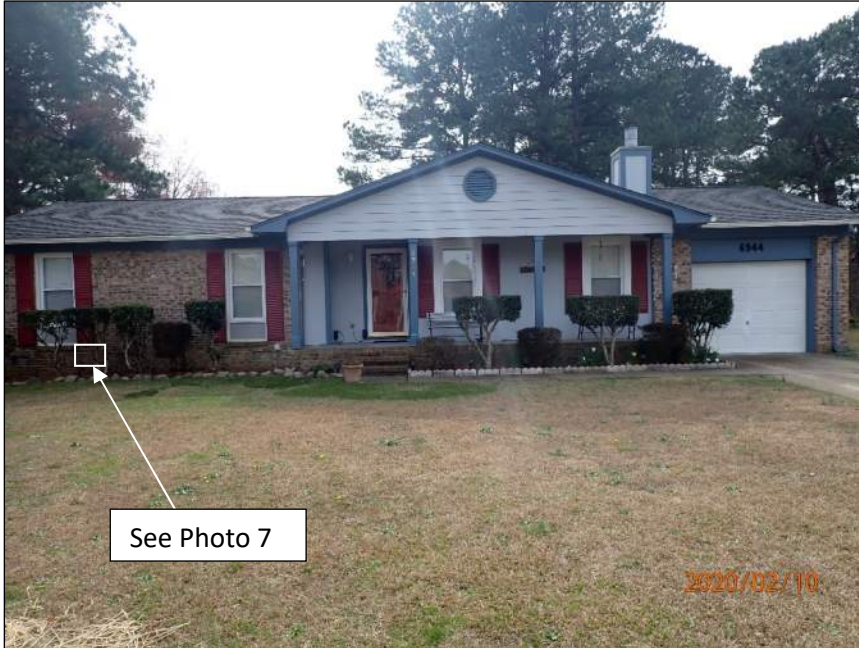
Photo 1 Area of residence observed – front elevation
