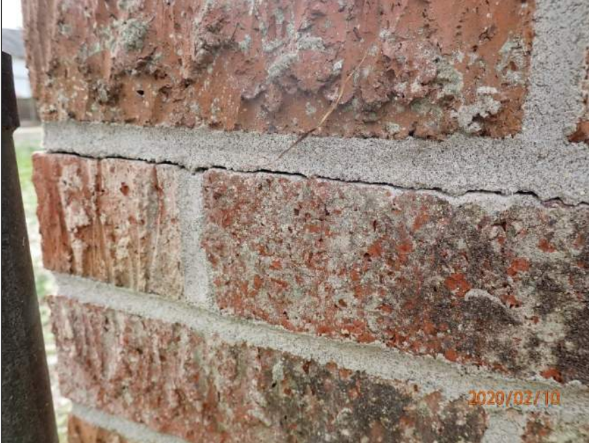
Photo 9 Horizontal crack
