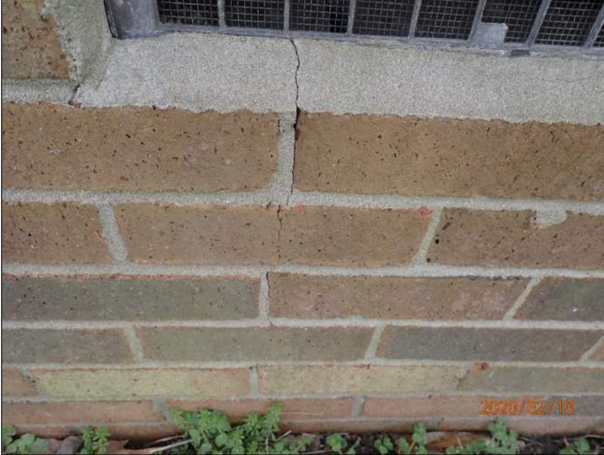
Photo 9 Vertical crack
