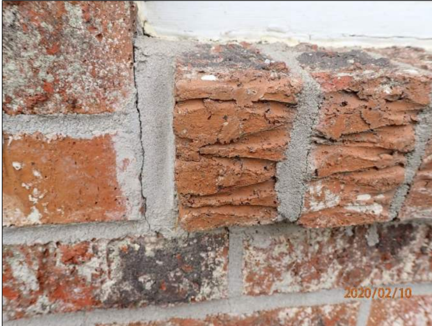
Photo 13 Vertical crack
