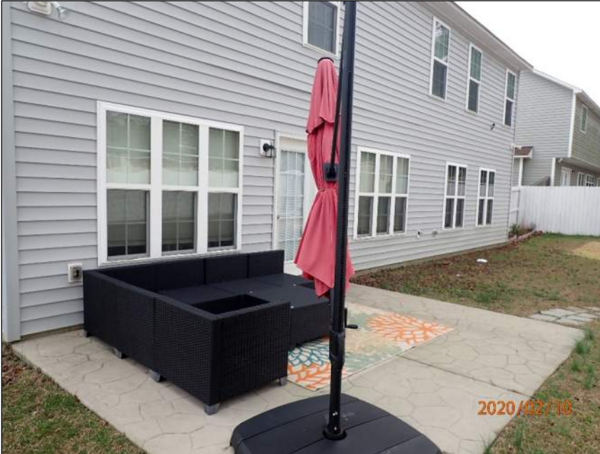
Photo 3 Area of residence observed – rear elevation
