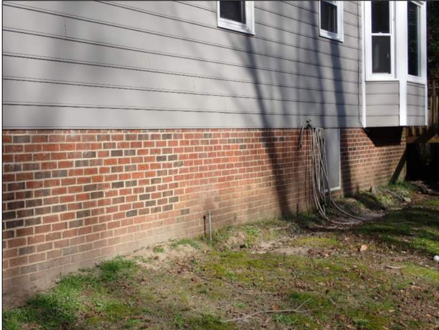
Photo 3 Area of residence observed – rear elevation (observed from outside fence)
