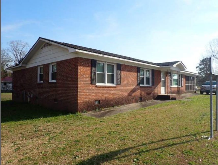
Photo 1 Area of residence observed – front elevation
