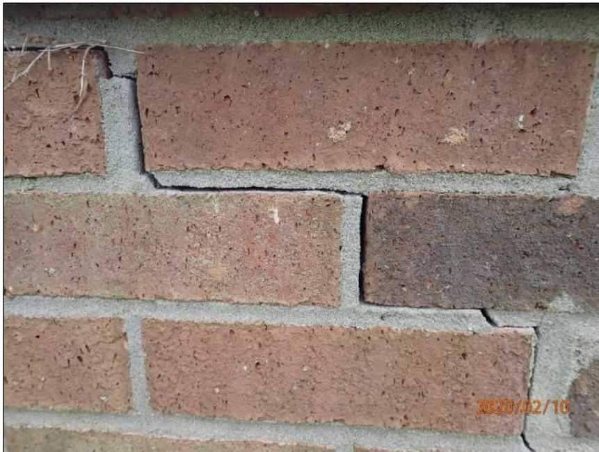
Photo 8 Step crack
