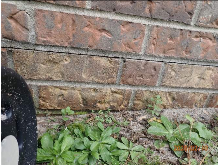
Photo 13 Horizontal crack
