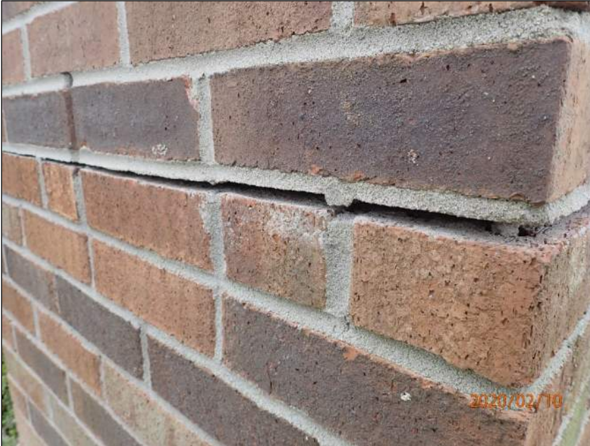
Photo 17 Horizontal crack
