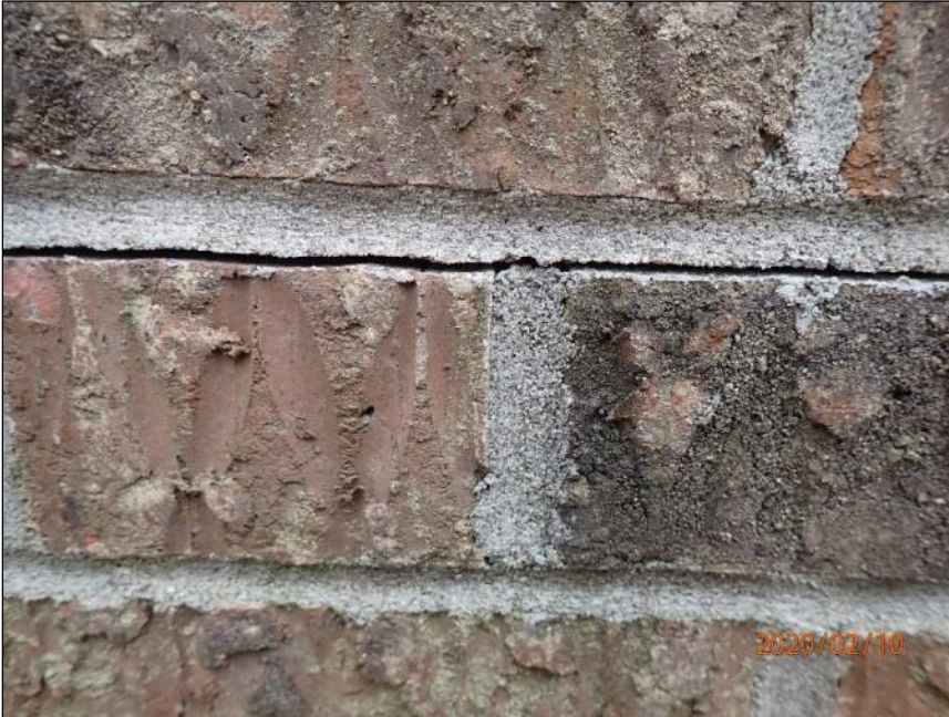
Photo 7 Horizontal crack
