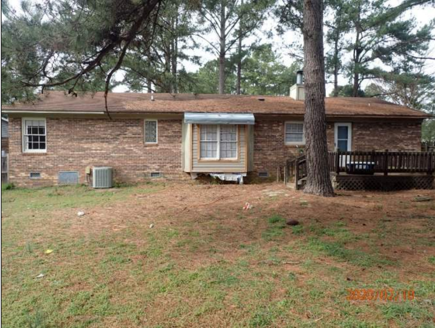
Photo 3 Area of residence observed – rear elevation
