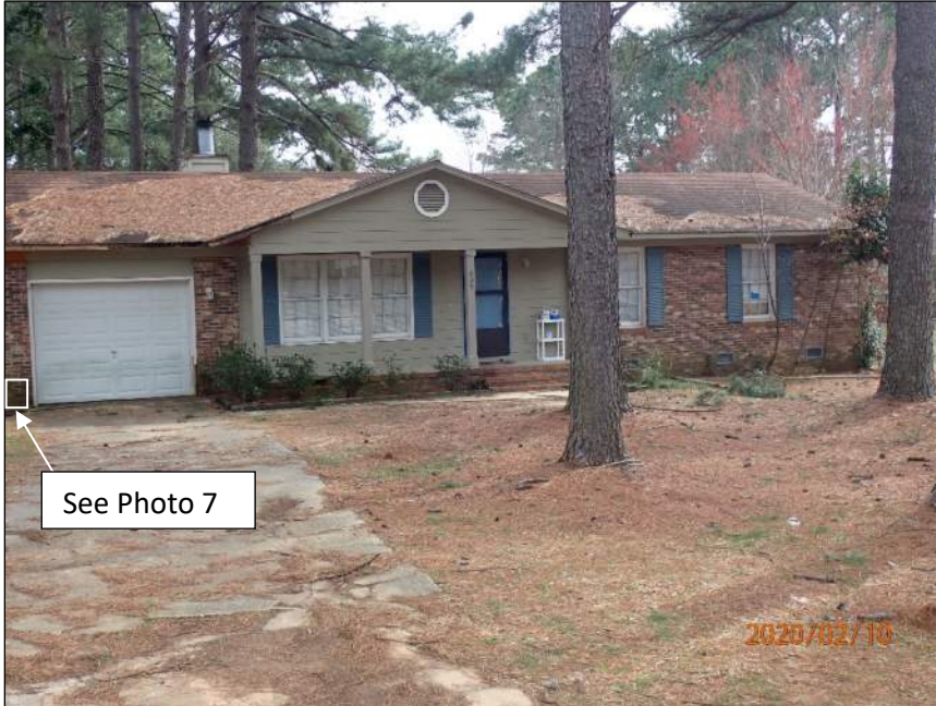
Photo 1 Area of residence observed – front elevation
