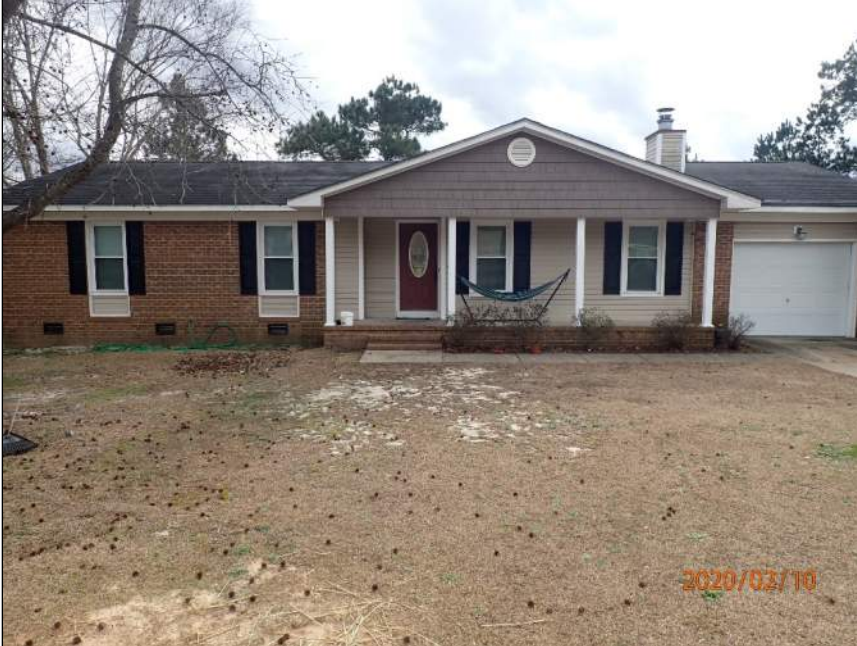
Photo 1 Area of residence observed – front elevation
