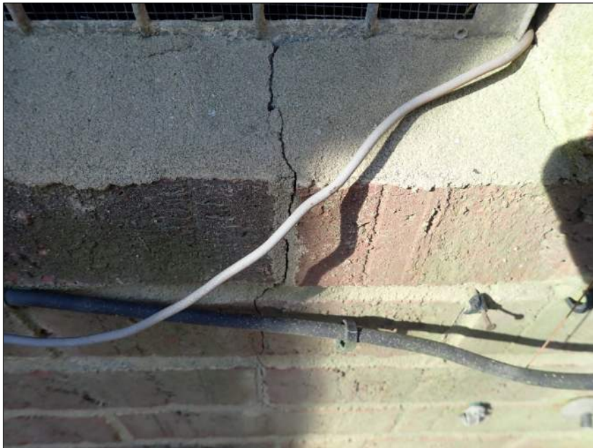
Photo 10 Vertical crack
