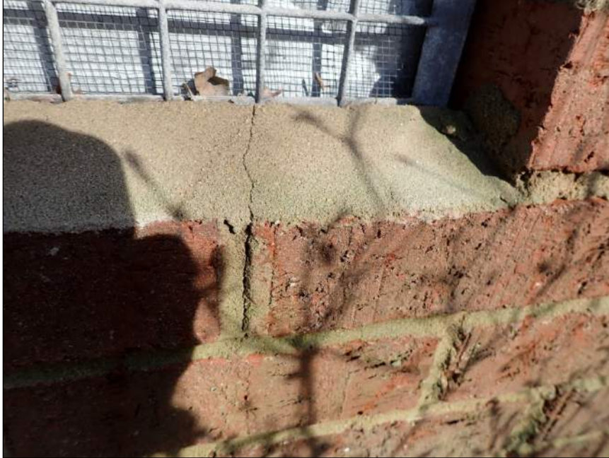
Photo 11 Vertical crack
