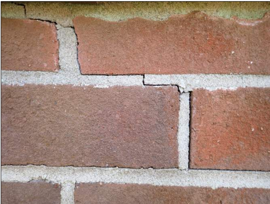
Photo 10 Step crack
