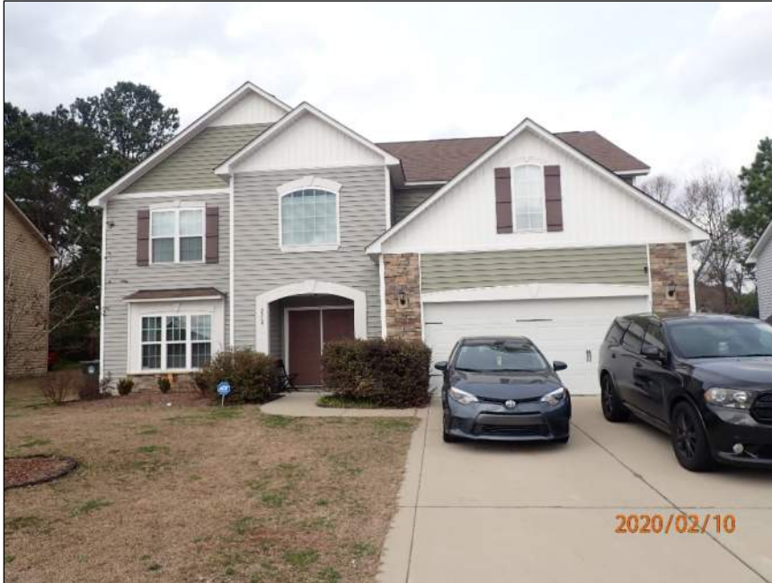
Photo 1 Area of residence observed – front elevation
