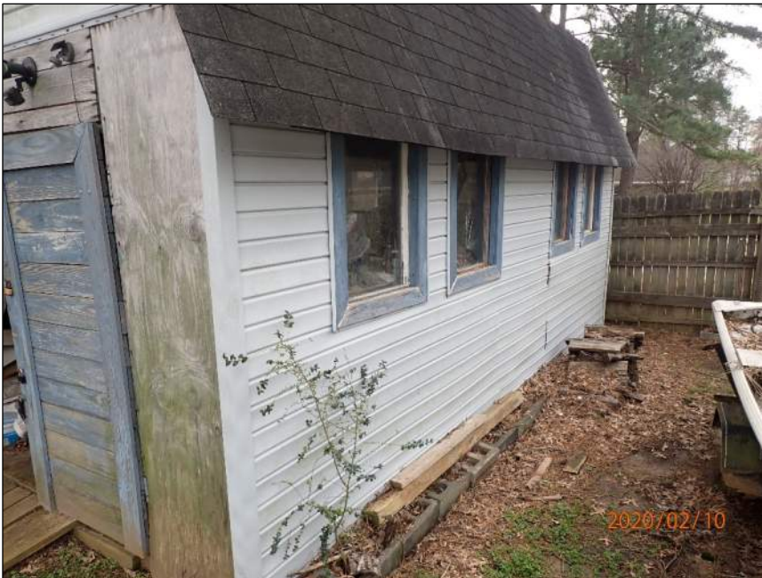
Photo 2 Area of structure observed
