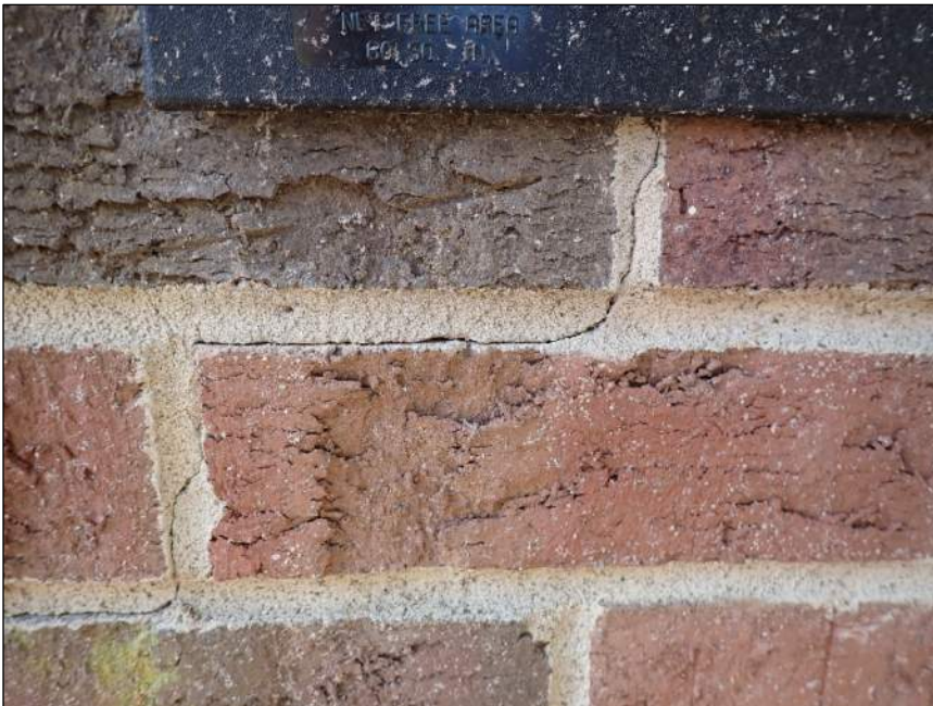
Photo 8 Step crack
