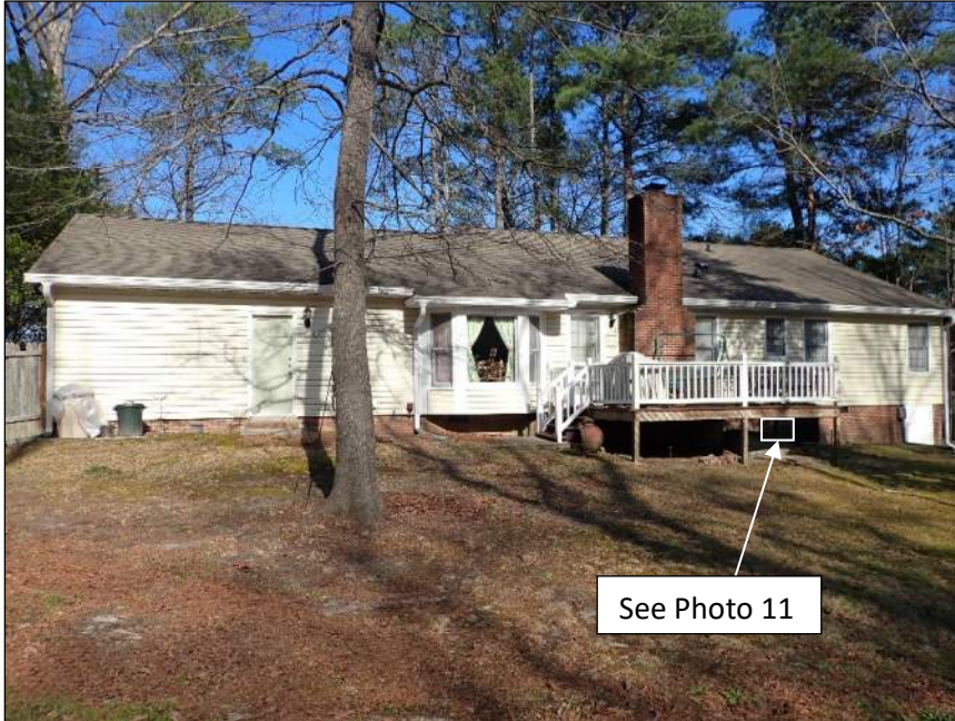
Photo 3 Area of residence observed – rear elevation
