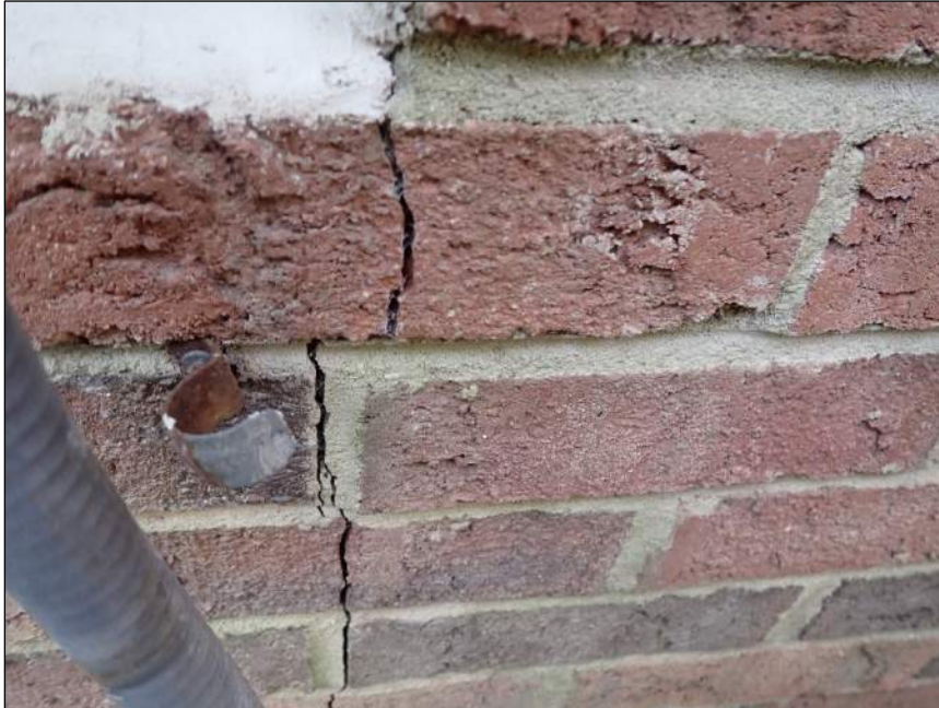
Photo 7 Vertical crack
