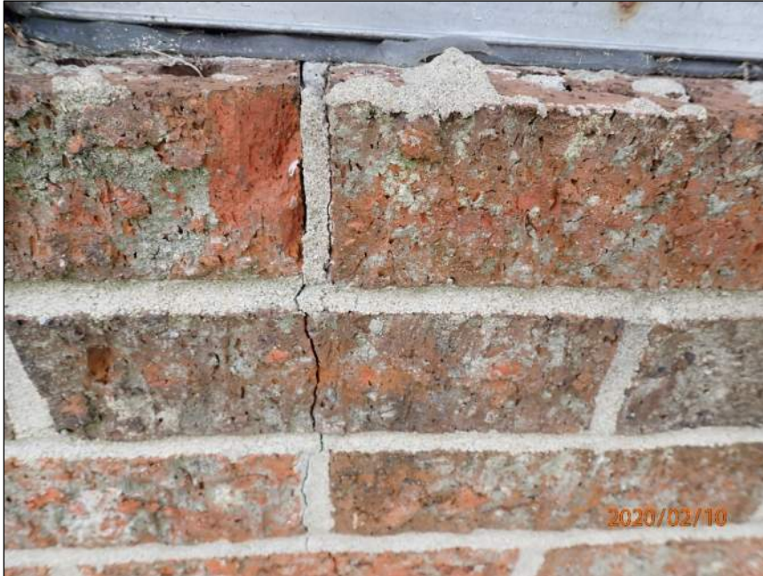
Photo 11 Vertical crack
