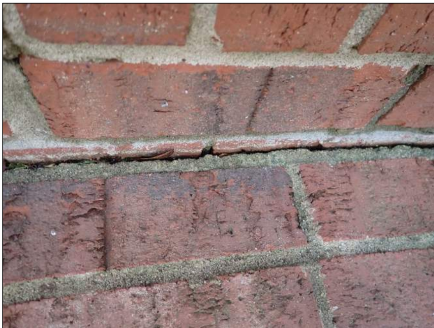
Photo 8 Separation crack
