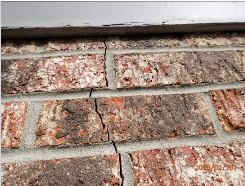
Photo 14 Vertical crack
