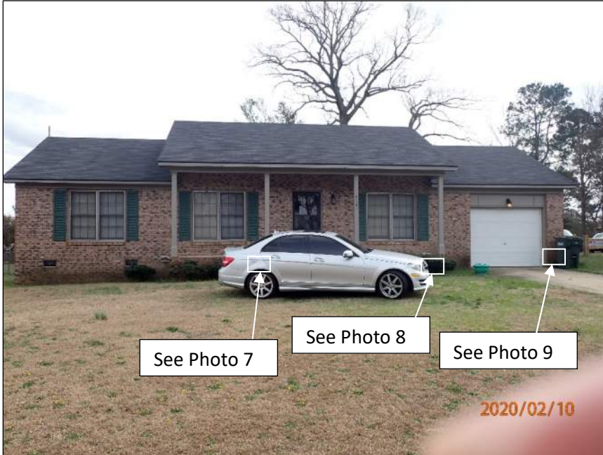
Photo 1 Area of residence observed – front elevation
