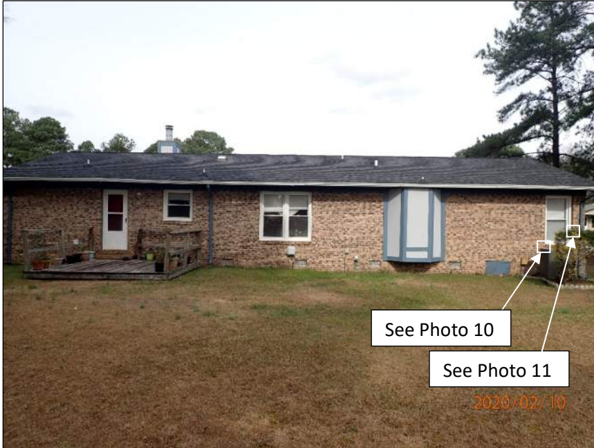
Photo 3 Area of residence observed – rear elevation
