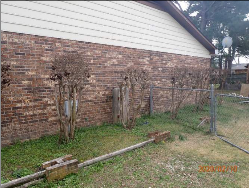
Photo 5 Area of residence observed – side elevation (partial)
