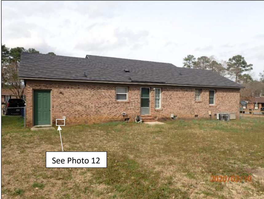
Photo 3 Area of residence observed – rear elevation
