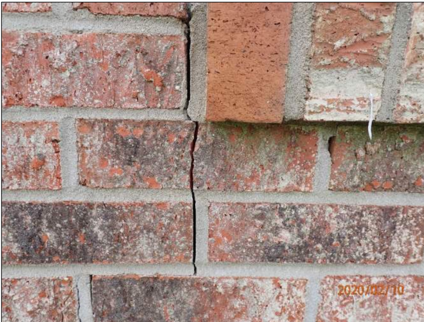
Photo 10 Vertical crack
