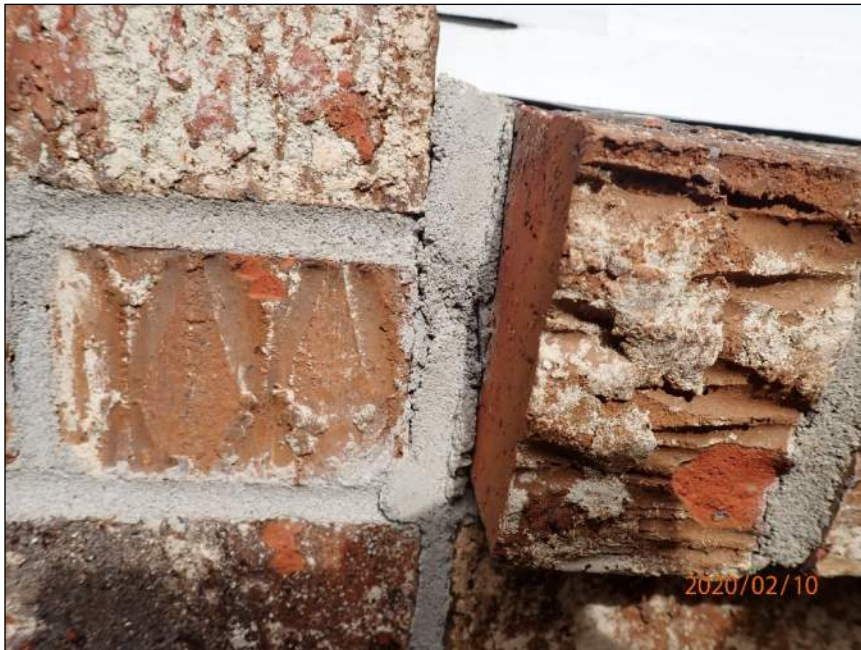
Photo 10 Vertical crack
