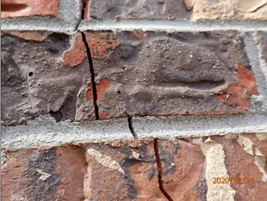
Photo 11 Vertical crack
