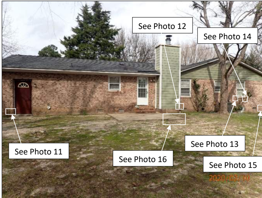
Photo 3 Area of residence observed – rear elevation
