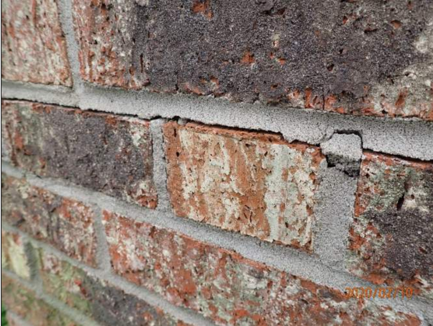
Photo 13 Horizontal crack
