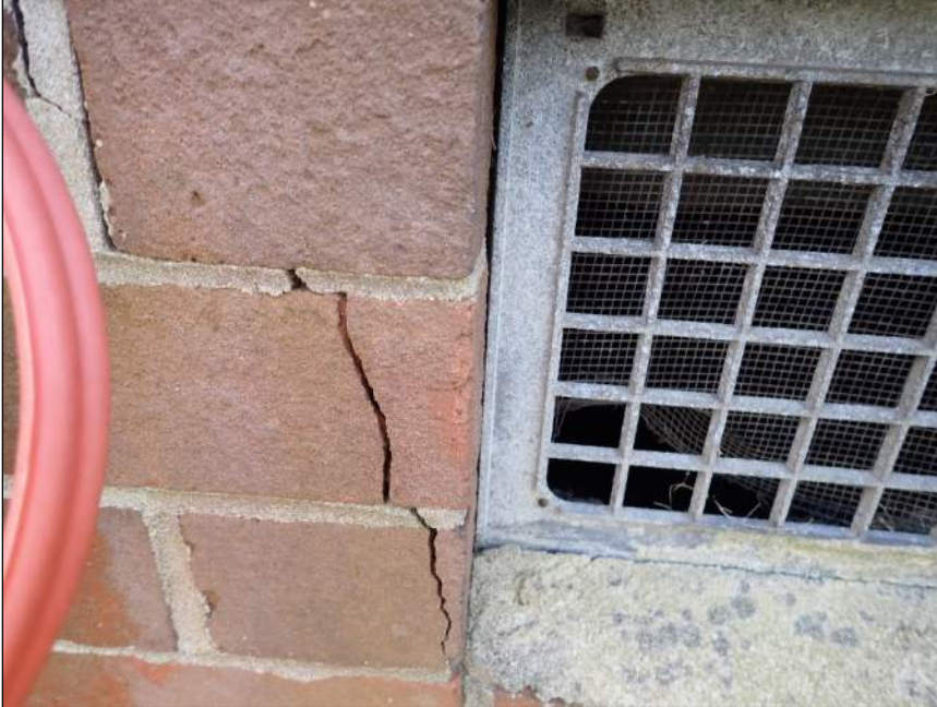
Photo 9 Step crack
