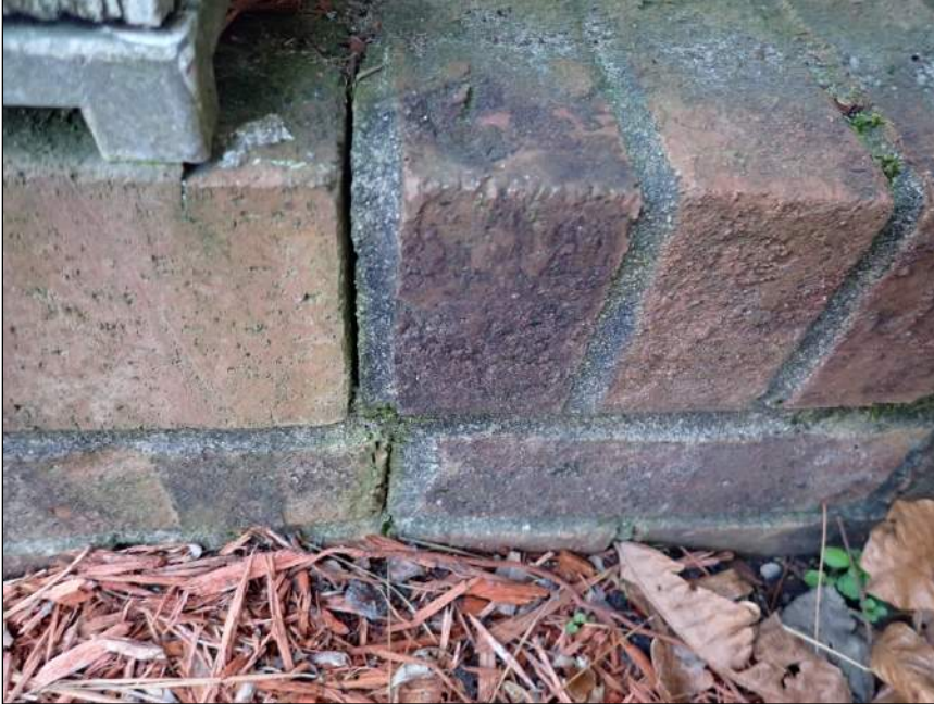
Photo 7 Vertical crack
