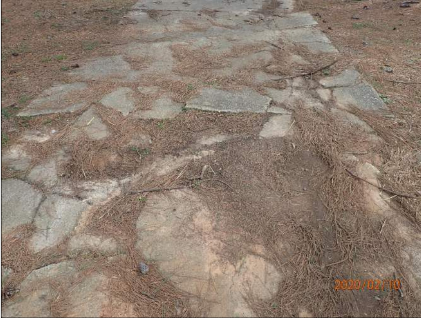
Photo 5 Cracks in concrete driveway
