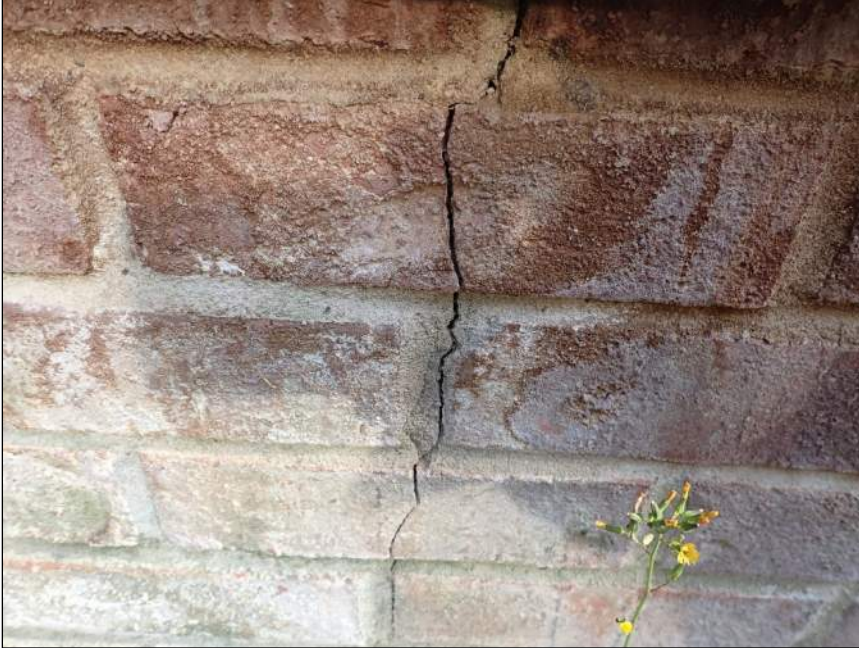
Photo 9 Vertical crack
