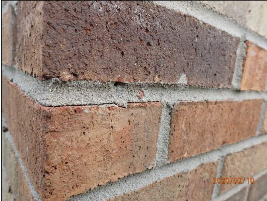
Photo 19 Horizontal crack
