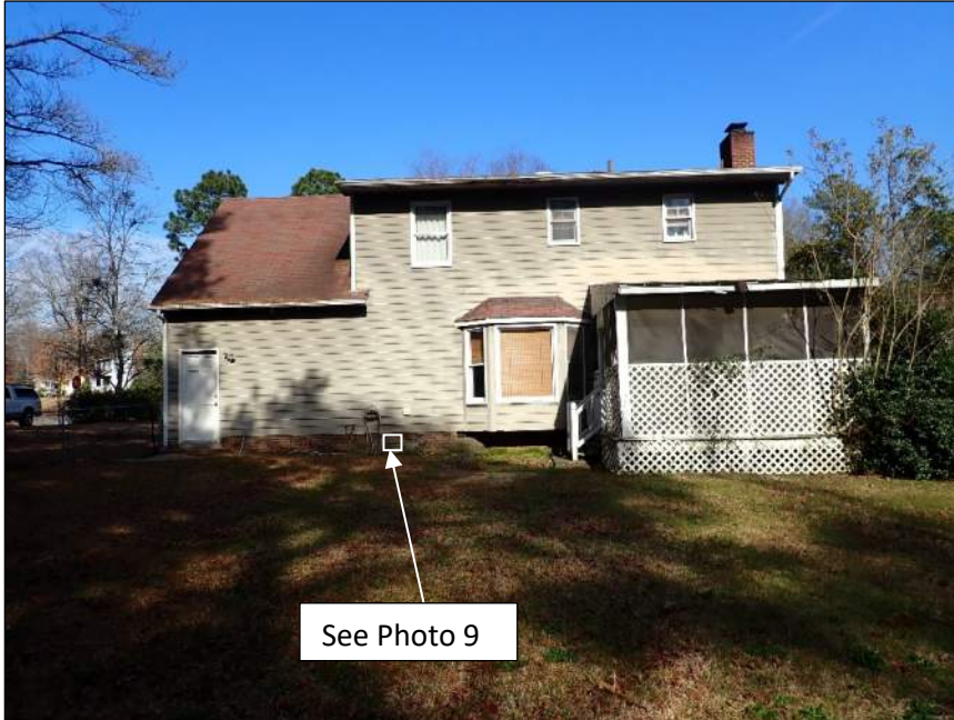
Photo 3 Area of residence observed – rear elevation
