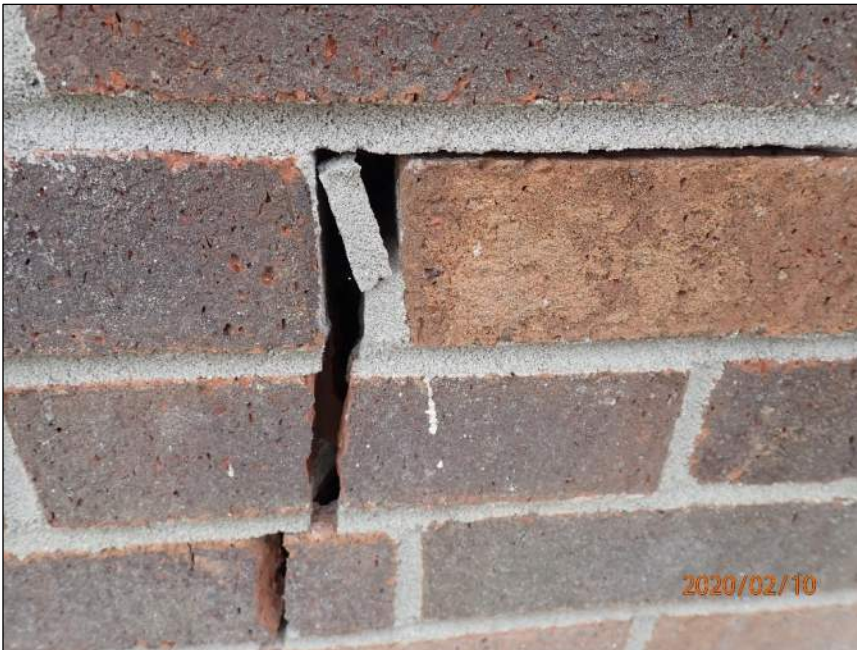
Photo 16 Step crack
