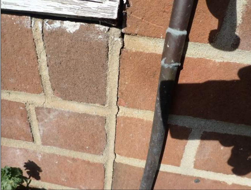
Photo 15 Separation crack
