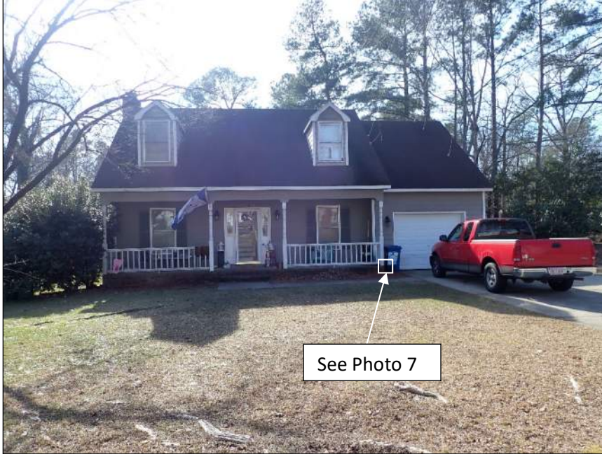
Photo 1 Area of residence observed – front elevation
