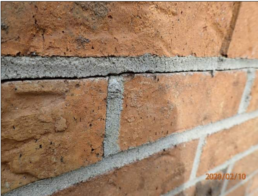
Photo 8 Horizontal crack
