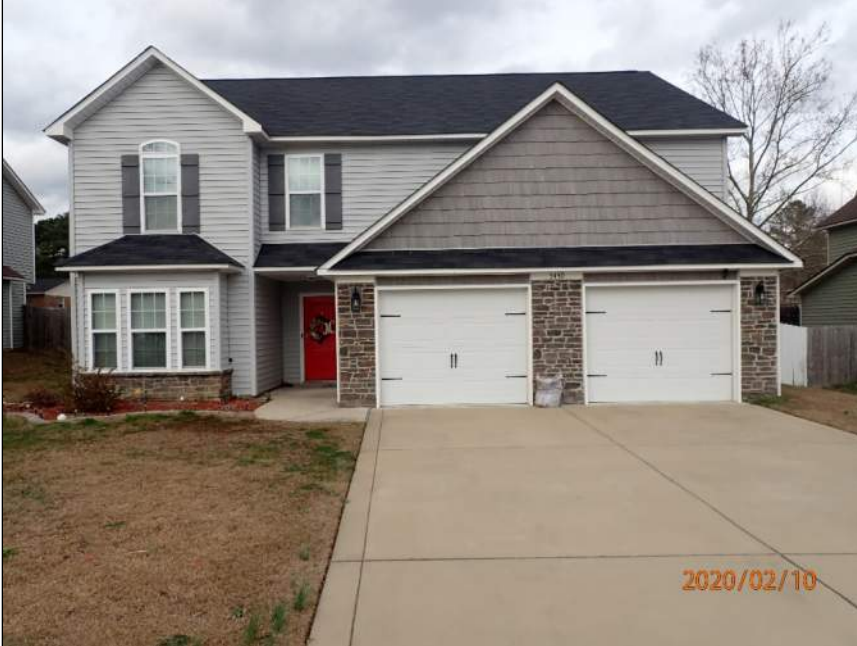
Photo 1 Area of residence observed – front elevation
