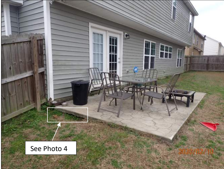
Photo 3 Area of residence observed – rear elevation
