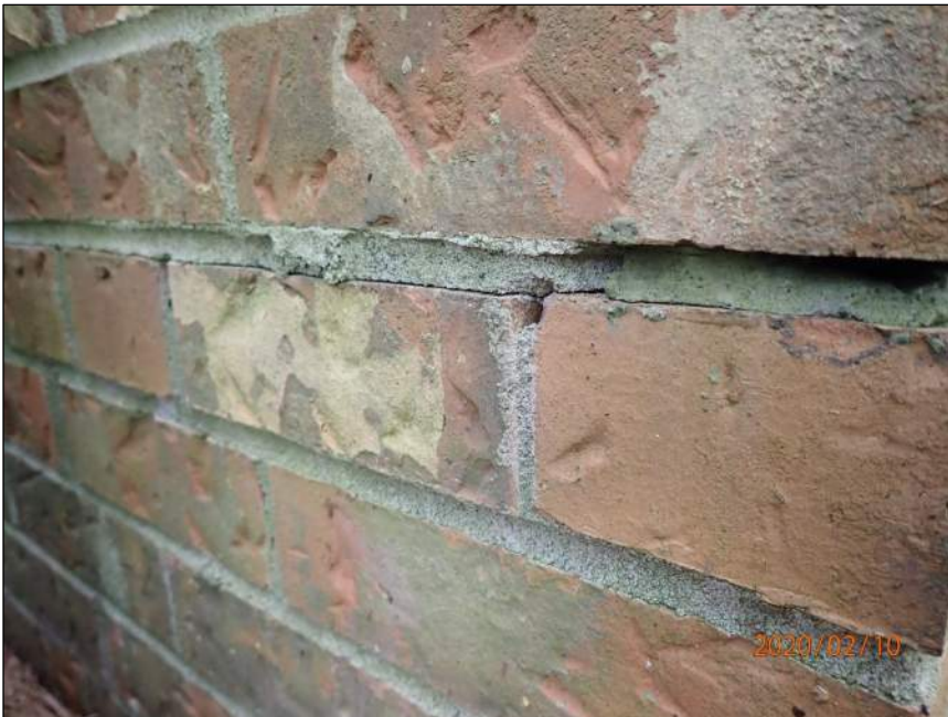
Photo 8 Horizontal crack
