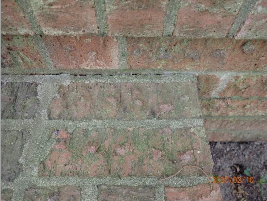
Photo 7 Separation crack
