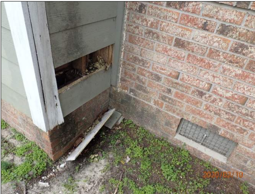
Photo 12 Missing siding
