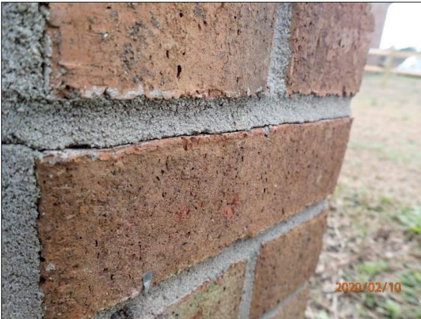
Photo 14 Horizontal crack
