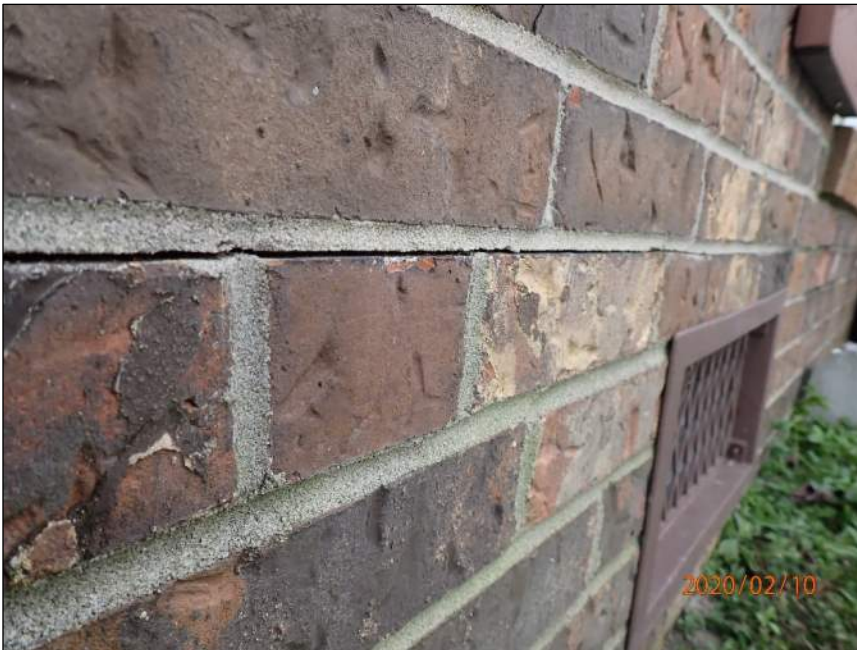
Photo 8 Horizontal crack
