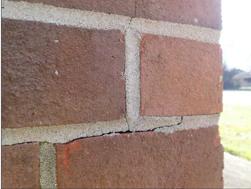
Photo 11 Step crack
