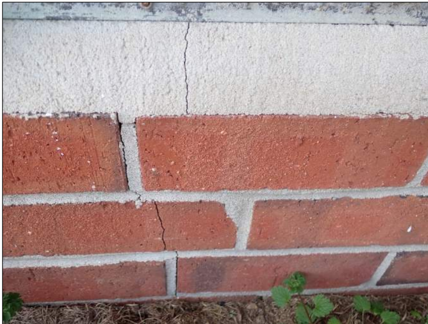
Photo 12 Step crack
