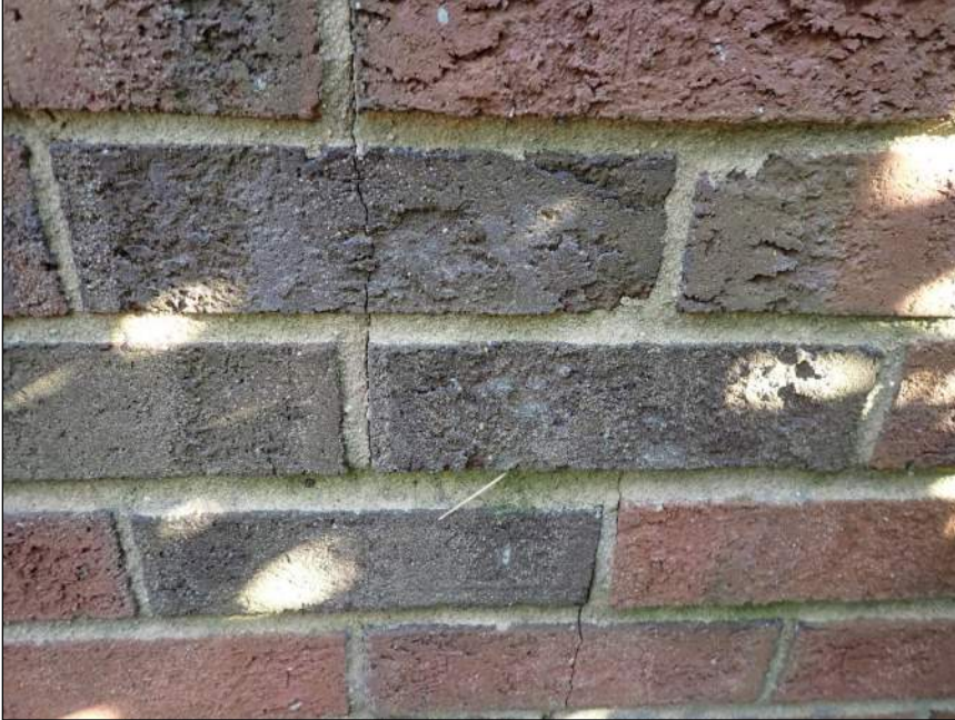
Photo 11 Vertical crack
