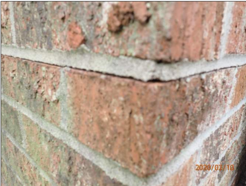
Photo 8 Horizontal crack
