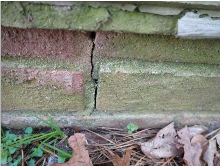
Photo 10 Vertical crack
