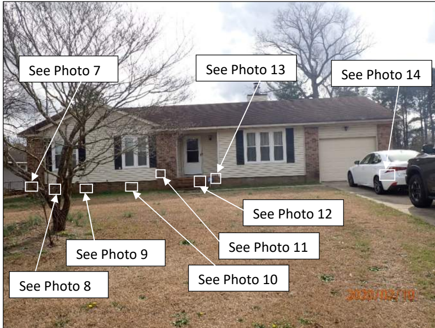
Photo 1 Area of residence observed – front elevation
