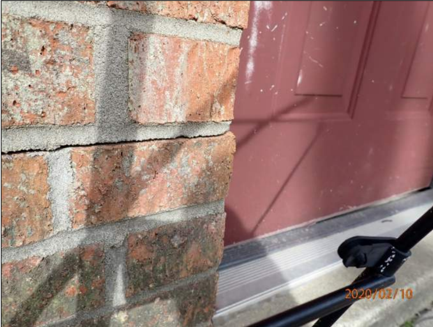
Photo 11 Horizontal crack
