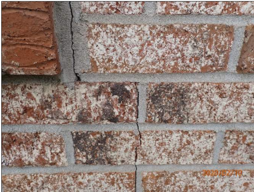
Photo 14 Vertical crack
