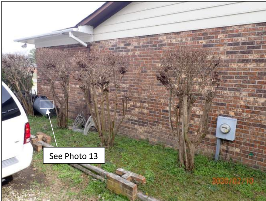
Photo 4 Area of residence observed – side elevation (partial)
