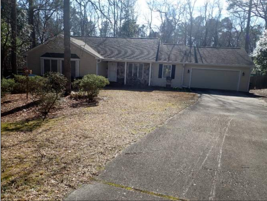
Photo 1 Area of residence observed – front elevation
