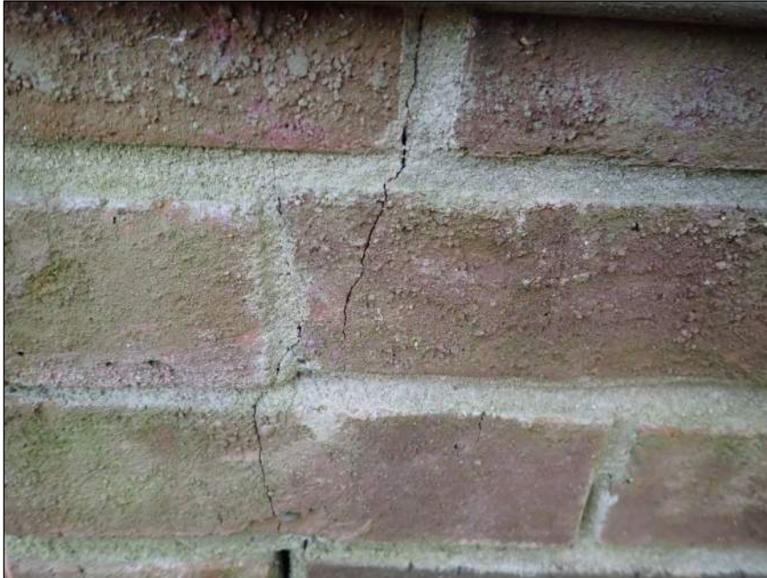
Photo 11 Vertical crack
