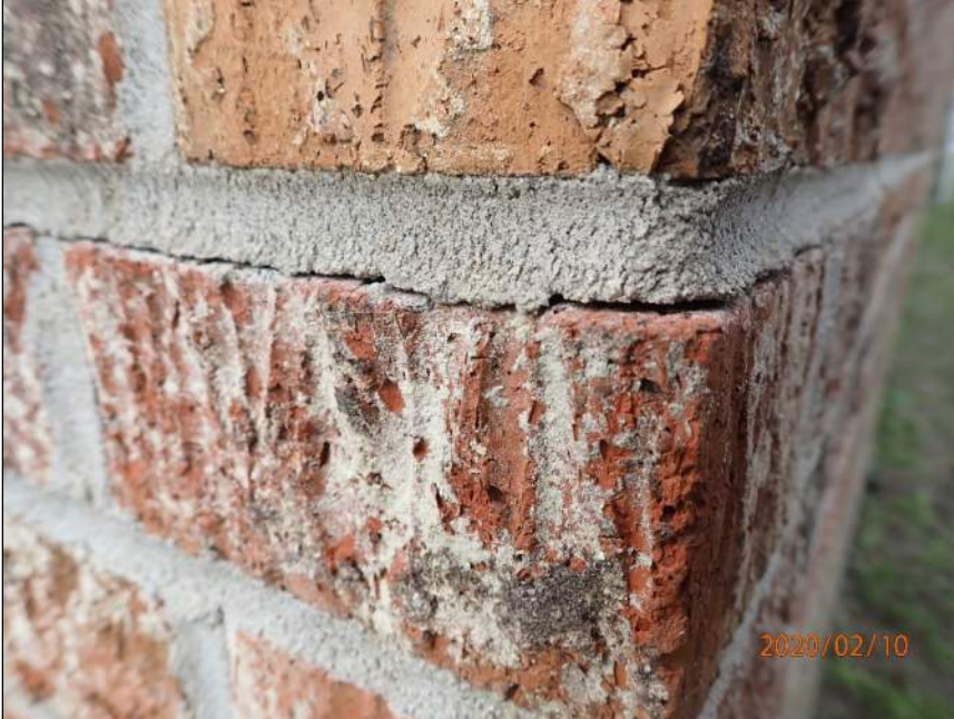
Photo 15 Horizontal crack
