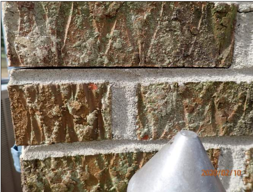
Photo 8 Horizontal crack
