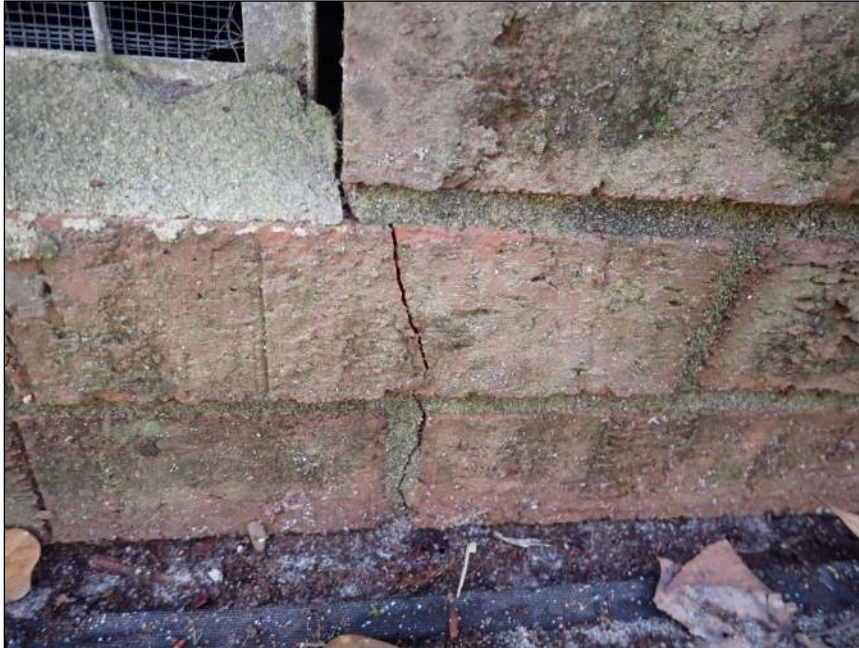
Photo 7 Vertical crack
